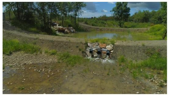
Fig. 1 - View of the inlet point and detention basin, and discharge into the infiltration basin
